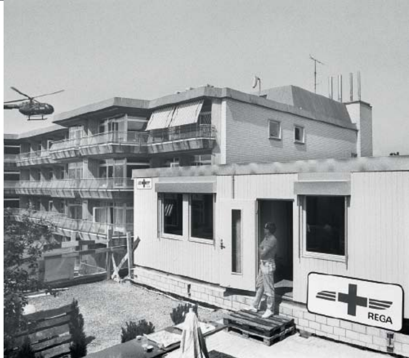
A transportable building on the hospital roof – the Zurich base in 1993.
